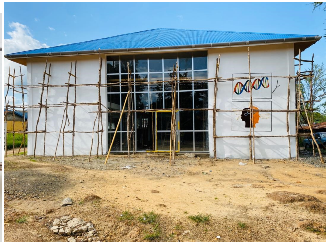
STEM and Biomedical Center Under Construction, Kenema, Sierra Leone, West Africa
